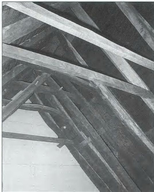
Plate 4 13th Century Base Cruck Roof at No 8 Bunyans Mead
